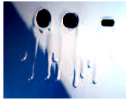
Removing paint runs
